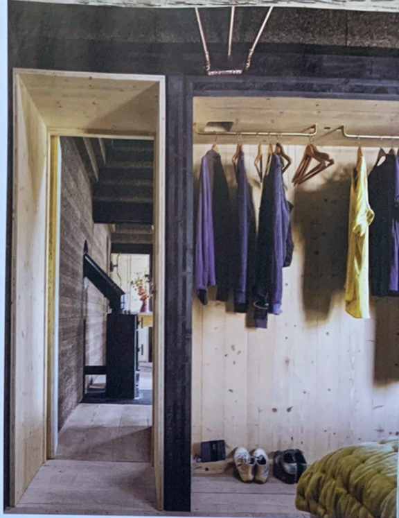
Fig 5: The cross walls lock the house together, with this one in the main bedroom opened out as a wardrobe. The floorboards, here and in the living room, are of American white oak
