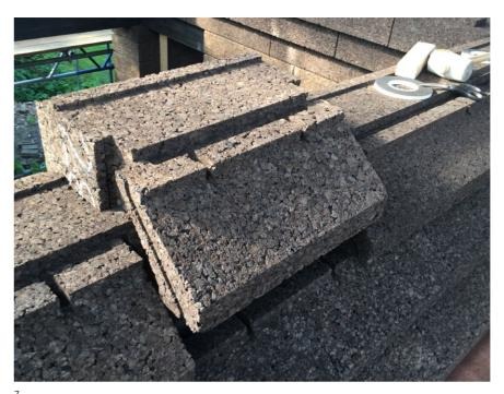
the assembly was correct, before being disassembled and shipped to site in Berkshire for re-assembly. This also served to test and demonstrate the readiness of the system for disassembly, a key part of the design allowing the cork blocks to be readily recovered for re-use at the end of the building's life.
